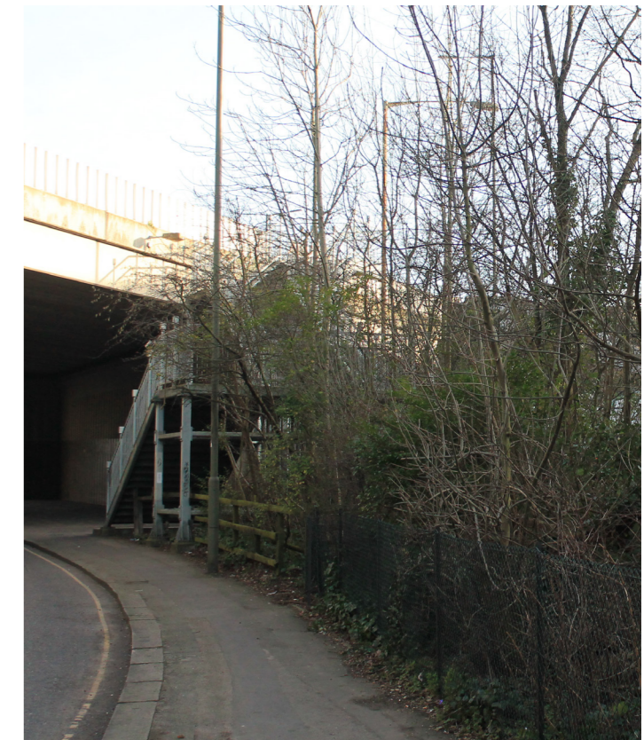
6 VIEW LOOKING EASTWARDS TOWARDS THE BRIDGE ON BUNNS LANE.
