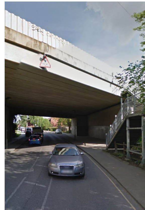
4 VIEW FROM BUNNS LANE TRAVELLING EAST
