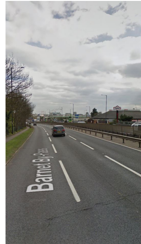
2 VIEW OF THE A1 TRAVELLING SOUTH
