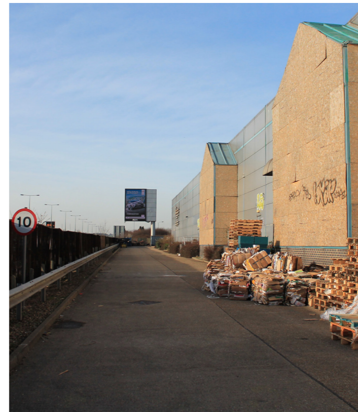
5 VIEW FROM THE EXISTING SERVICE ROAD (SOUTHERN FACADE) OF PENTAVIA RETAIL PARK FACING THE M1.
