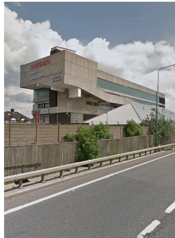
3 VIEW FROM THE M1 OF NISSAN GARAGE
