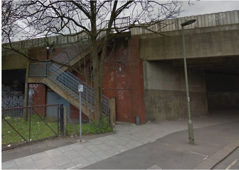
Existing stair East from A1
