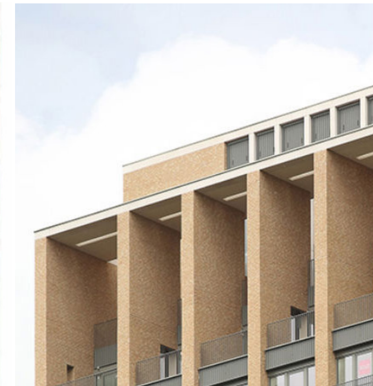
BRICK PIERS AND WHITE HORIZONTAL FRAME
