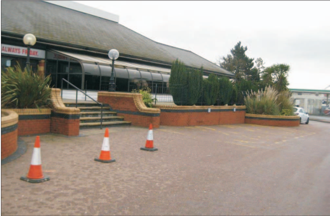
PHOTOGRAPH 3: View of Building B2
