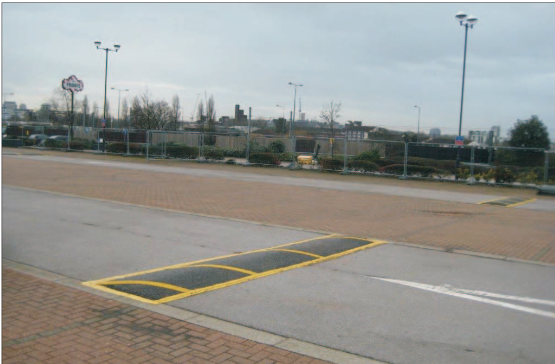
PHOTOGRAPH 4: View of Hardstanding
