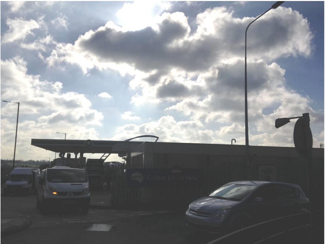
Figure 27: View of side elevation of BP petrol services to the south of the site.
