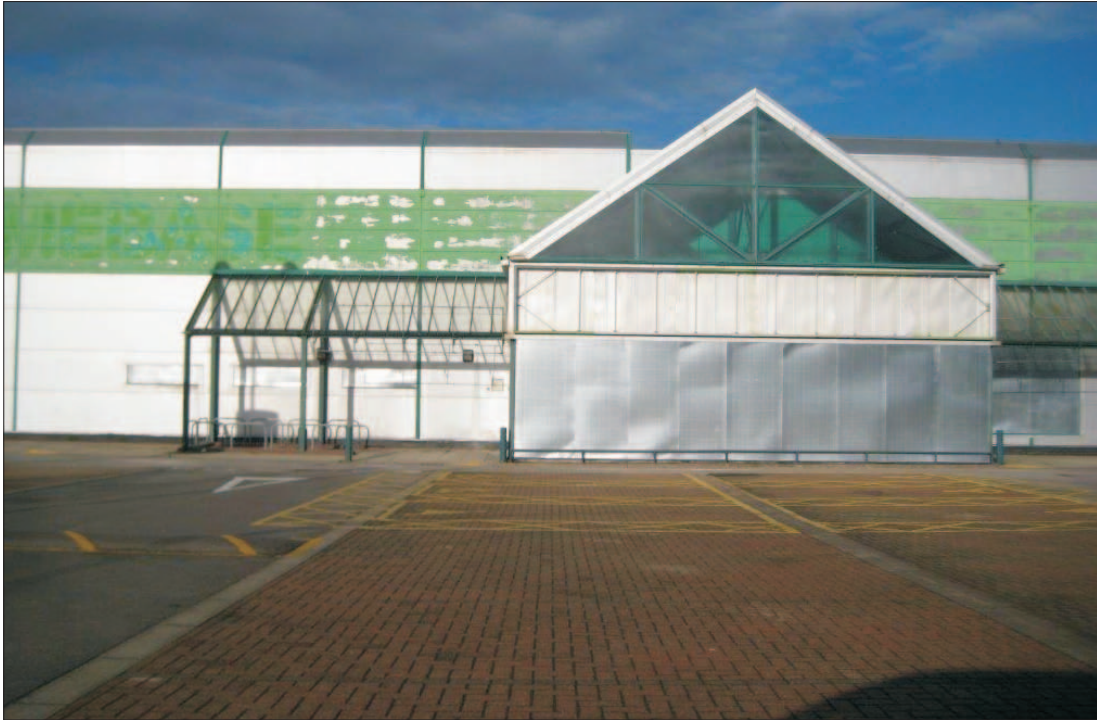
PHOTOGRAPH 1: View of Building B1
