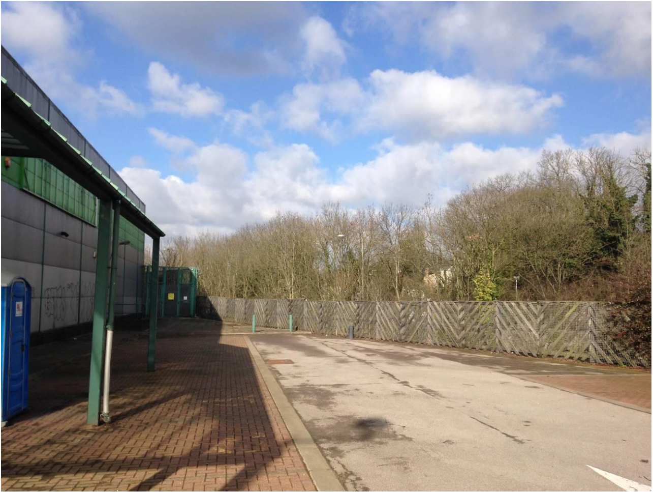
Figure 22: Detail view of fencing and landscaping to the north eastern boundary.
