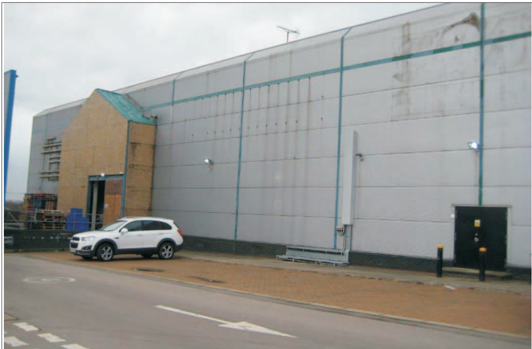
PHOTOGRAPH 2: View of Building B1
