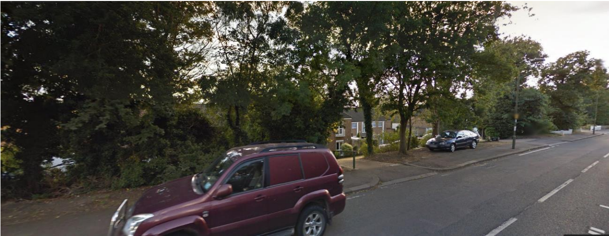
Figure 33: View from Featherstone House, Wise Lane, towards the Site.
